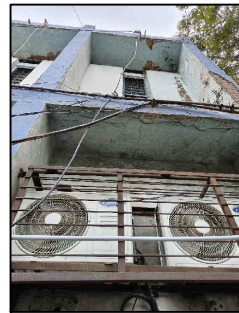
structural Patch repairs Required
