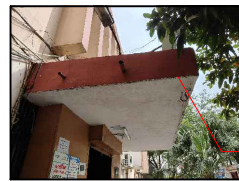
structural Patch repairs Required & Plaster Required
