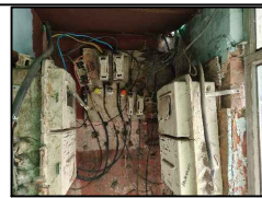
Electrical Main DB Panel to be replaced
