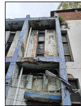
Windows to be Replaced & structural Patch repairs Required
