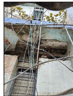
Windows to be Replaced & structural Patch repairs Required & RW Pipes to be Replaced
