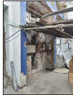
Wall Cracks to be repaired & Plaster required
