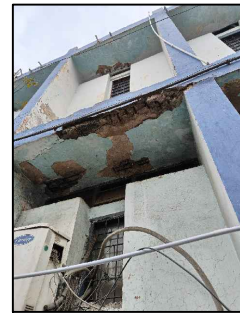
structural Patch repairs Required
