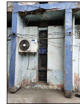
Windows to be Replaced & structural Patch repairs Required
