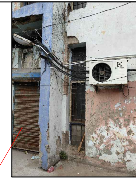
Wall Cracks to be repaired & Plaster required
